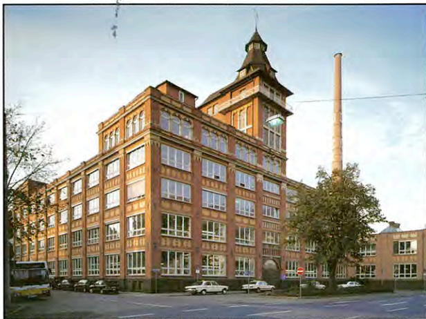
Friedr. Dick GmbH, altes Firmengebäude in Esslingen Former building in Esslingen
